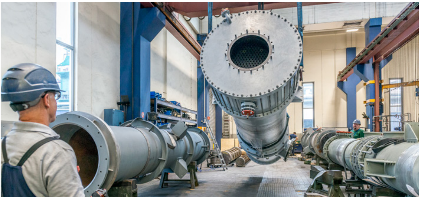
↑ Lifting of a DIABON® heat exchanger
